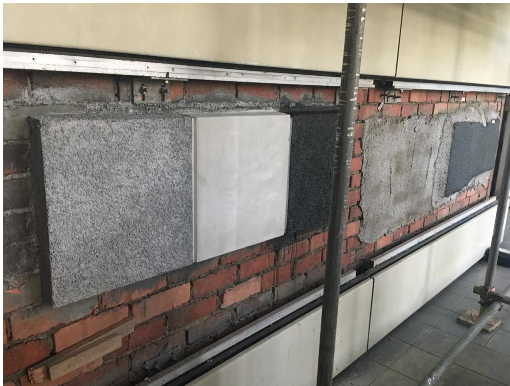
1 st from Left: Lighterm applied in a single application with a thickness of 40mm
