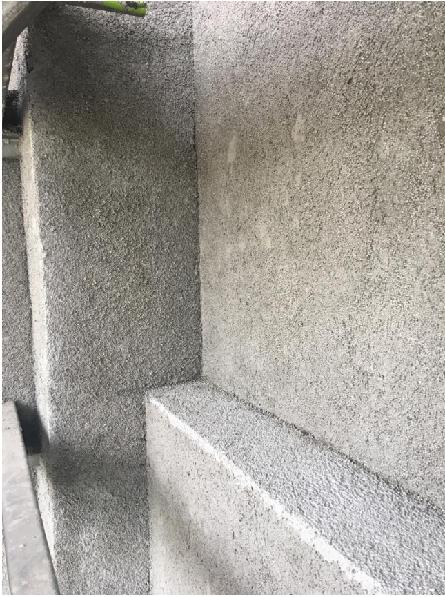
Perpendicular joint well coated
