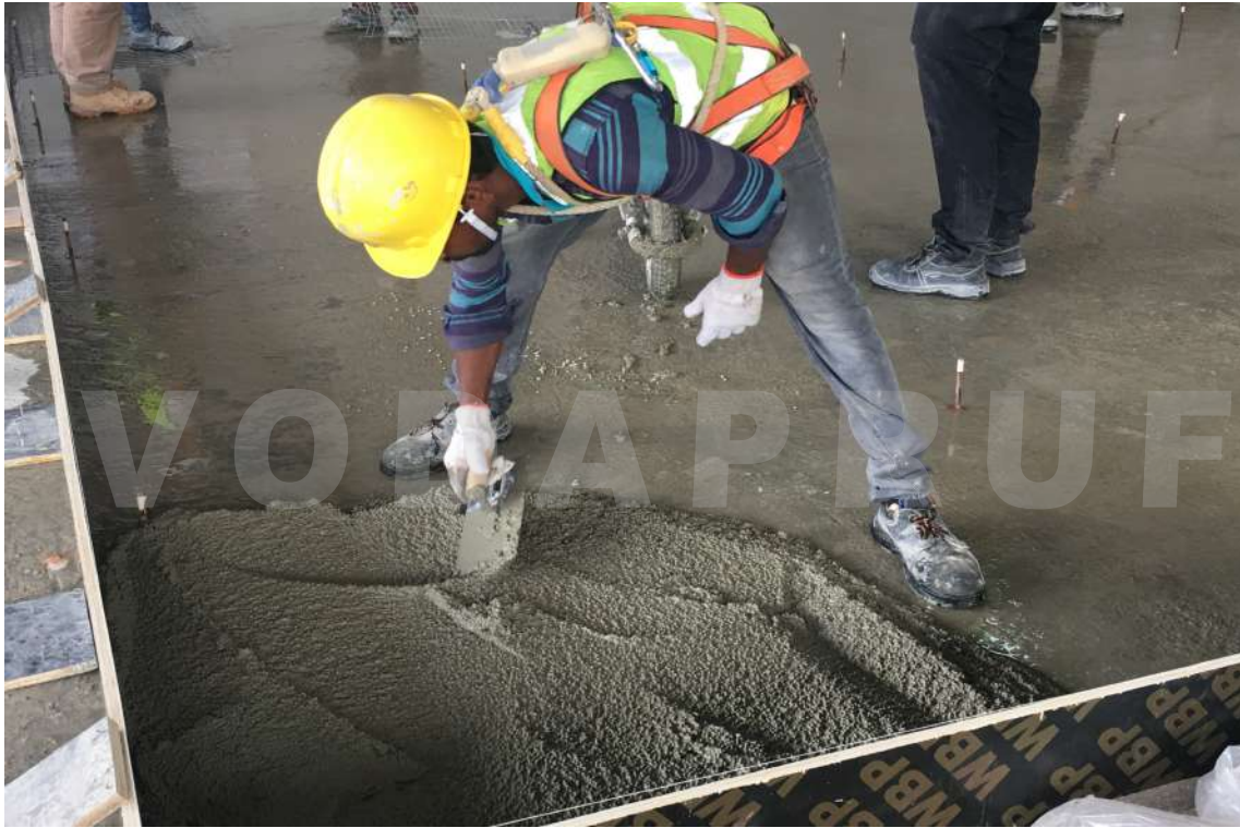
proper trowelling of LIGHATHERM screed
