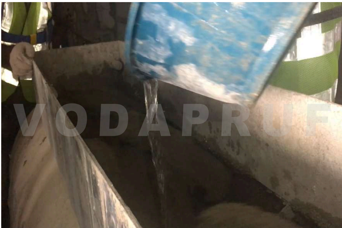
Water added according to ratio stipulated and mix for 5 minutes . No additional material required.
