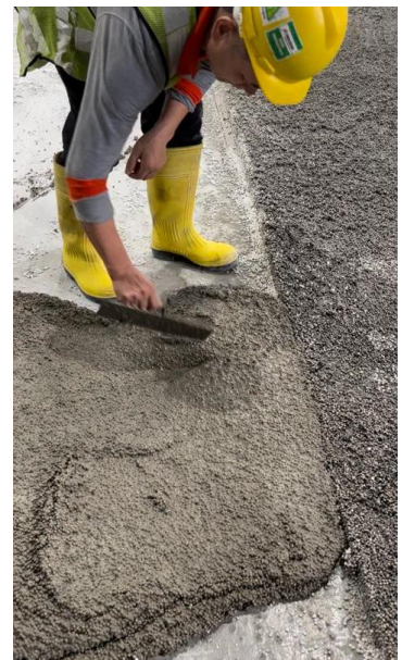
Picture above shown the polyfoam beads blend well with cement without segregation
