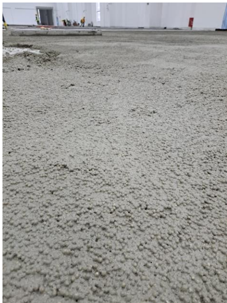
Picture above shown the polyfoam beads blend well with cement without segregation
