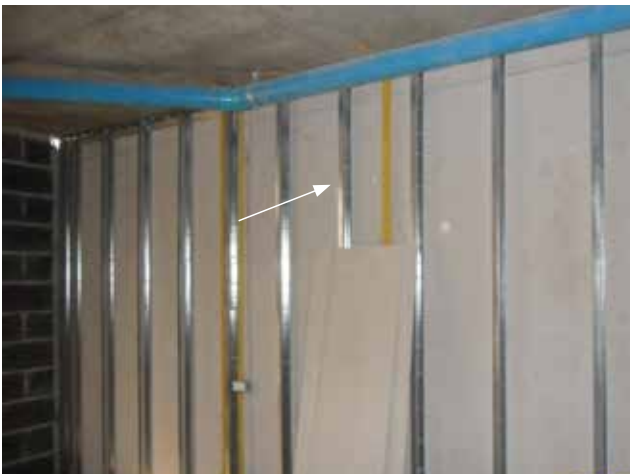
Installation of GI frame
