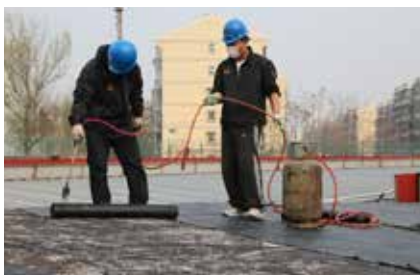
Waterproofing membrane application on Lightherm Screed
