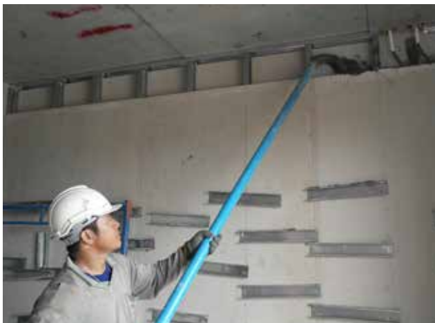
Infill of Lightherm into hollow section
