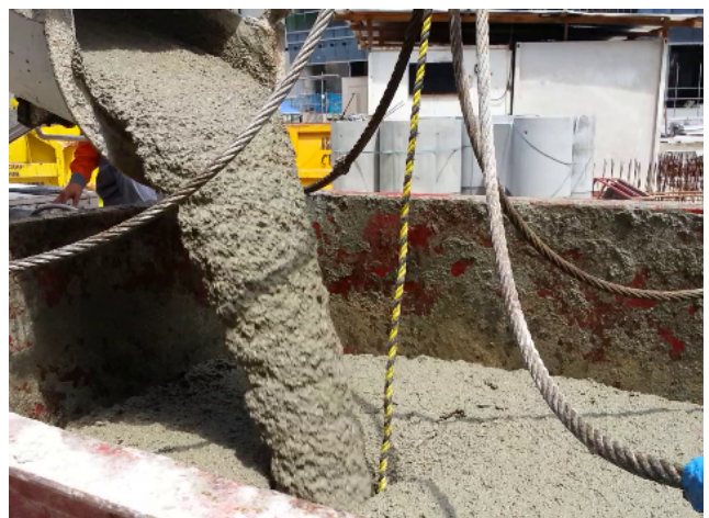
Pouring of Lightherm Screed
