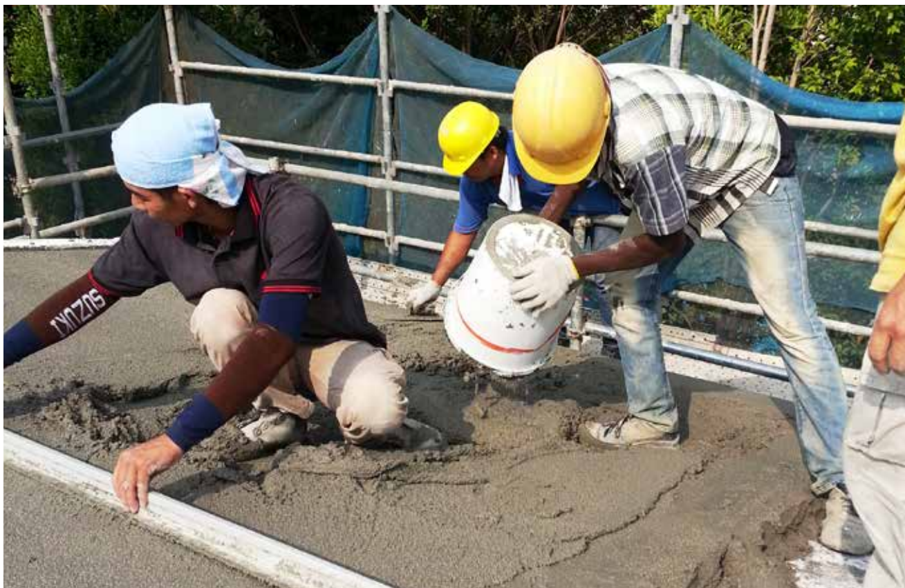
Lightherm Screed as roof insulation layer
