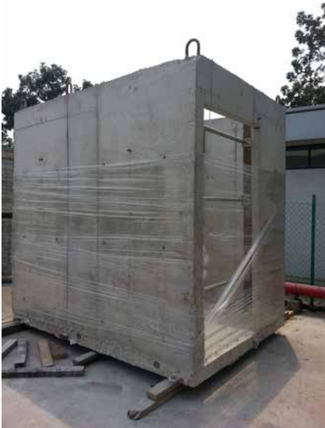
Density 1000kg/m 3 , achieved compressive strength of 7N/mm 2
