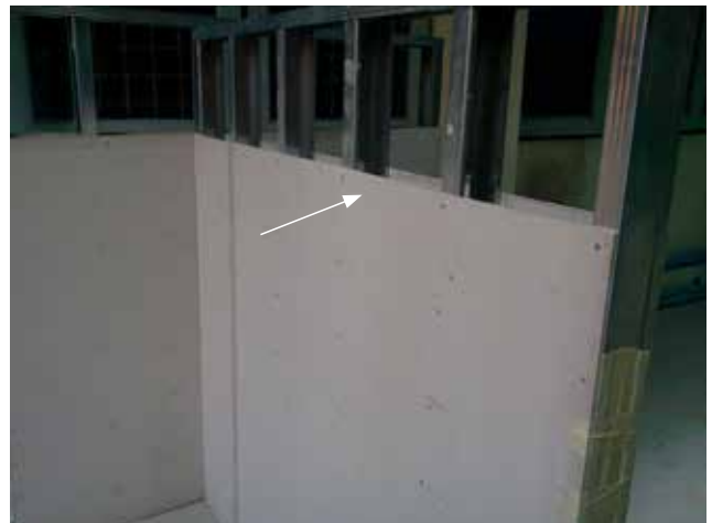
Installation of cement board
