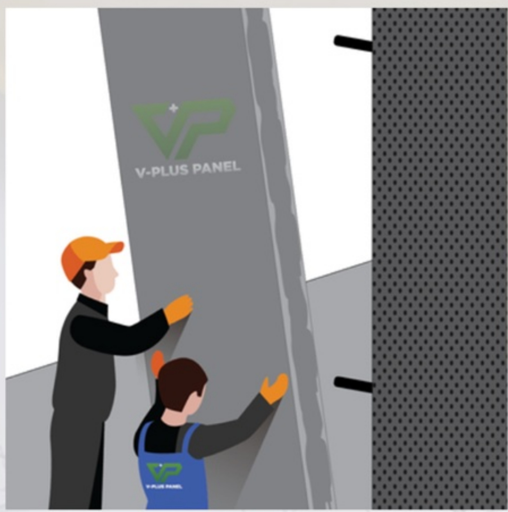
Install VPLUS Panel vertically attach to the column.
