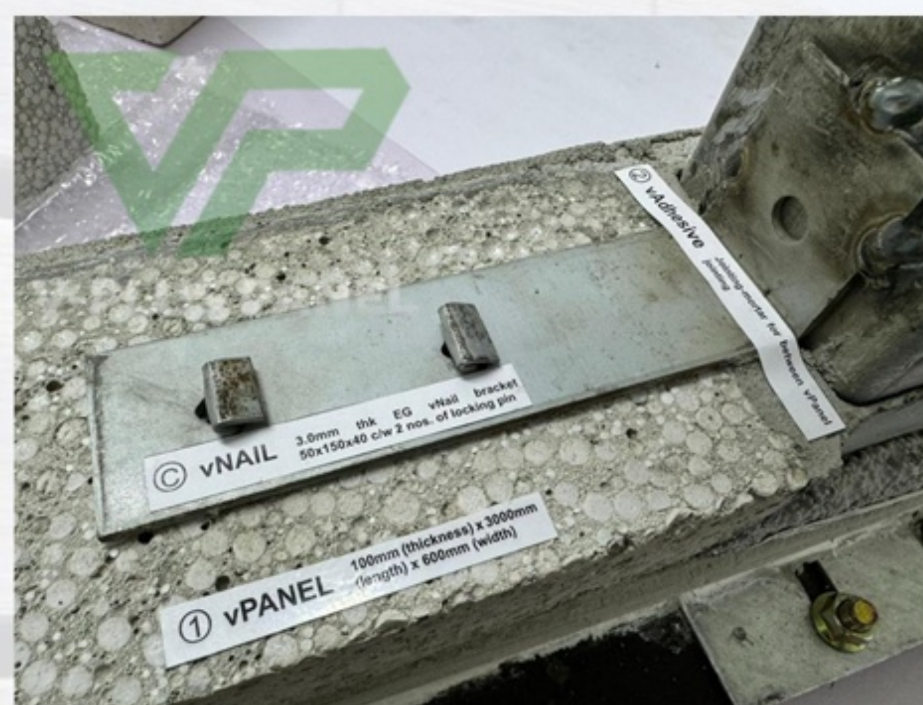
Typical design of vNAIL-Bracket and vNAIL Locking Pin
