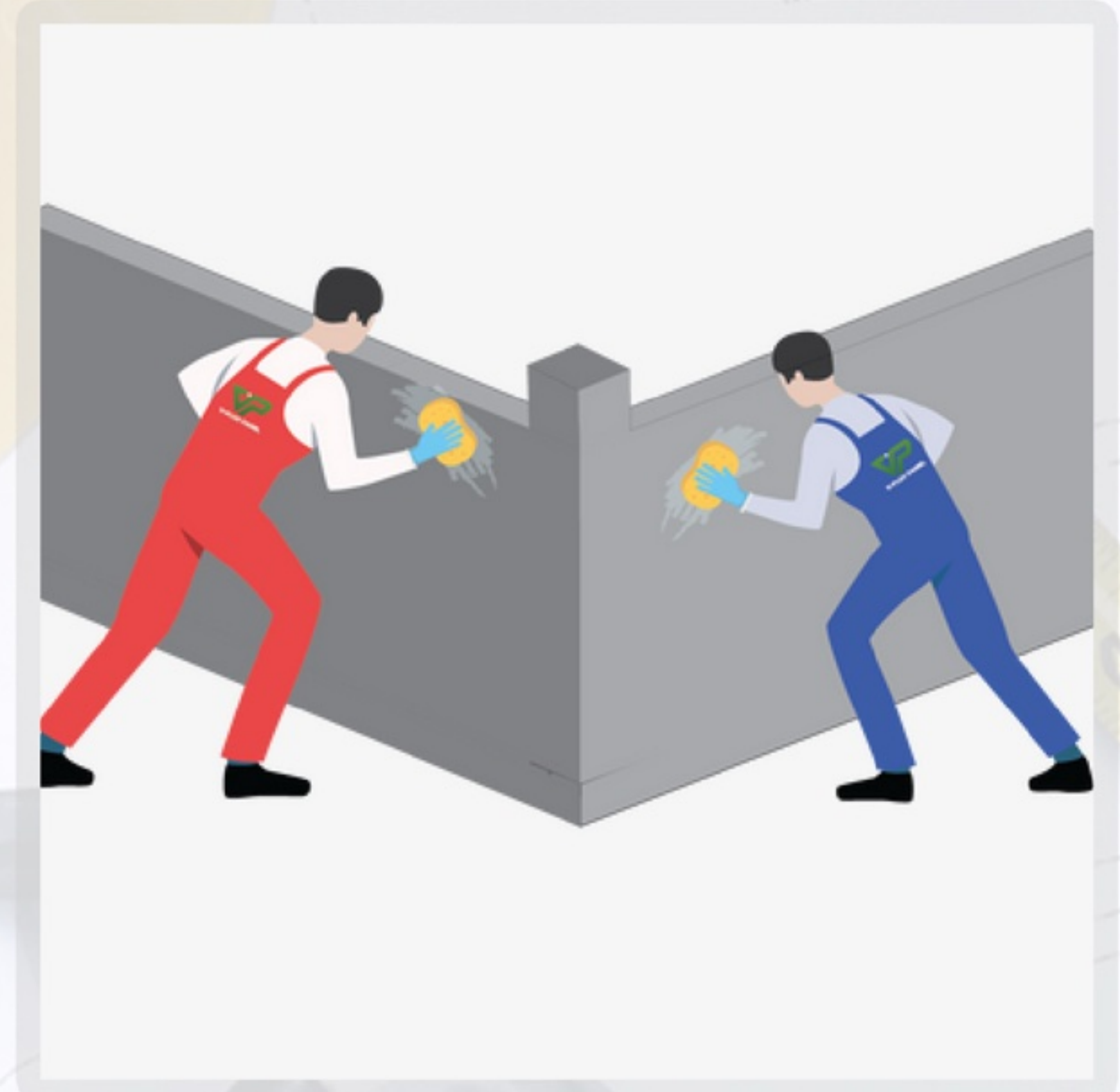
Apply skim coat to overall panel wall surface
