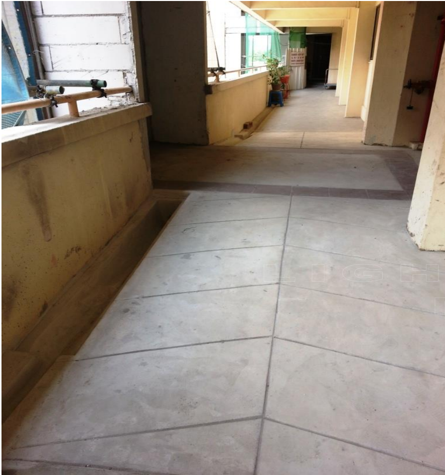
As lightweight screed of only 250kg/m 3 - Lift upgrading works for HDB @ Jurong East Street 13
