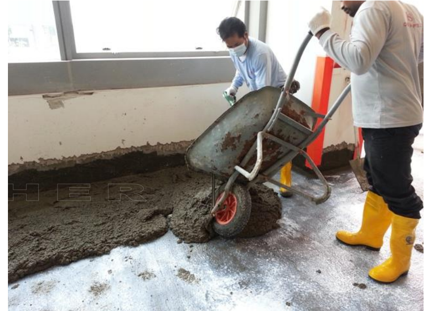
On site application
