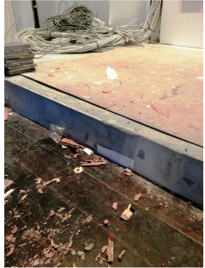
Insulation layer to prevent condensation -- Conservation Unit @ 136 & 138 Neil Road
