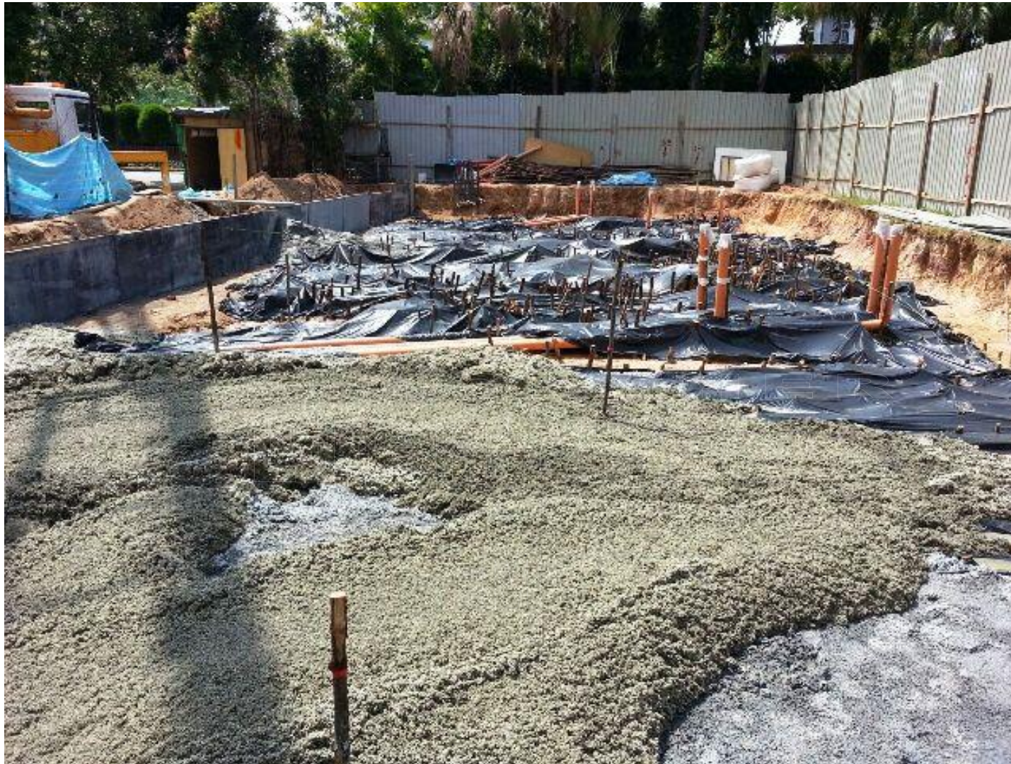
Filler before casting of ground floor slab - 90 Meyer Road
