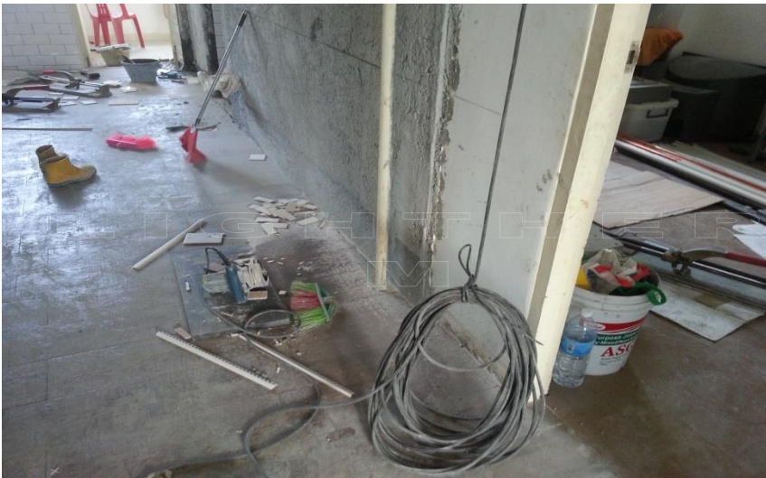
After tiles application
