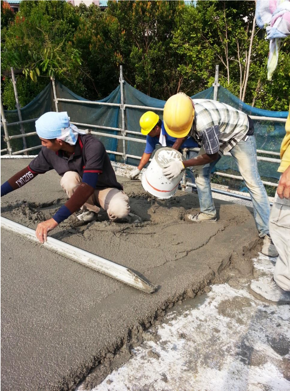
As roof insulation layer - Terrace House @ 19 Buckley Road
