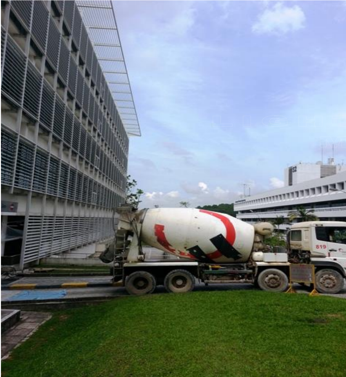
Material batched in concrete truck
