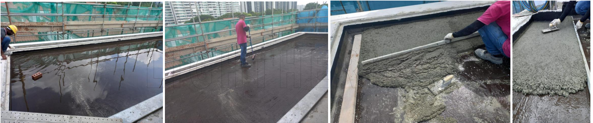
Insulation Methods : As lightweight Thermal Insulation Screed on Roof for various Residential & Commercial Buildings
