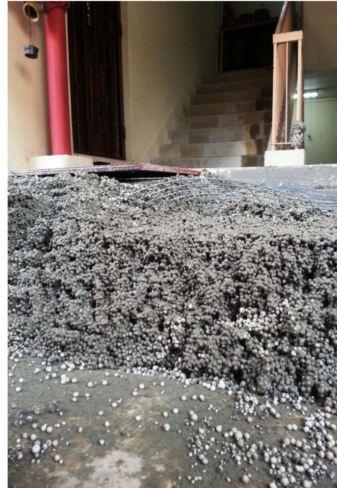
As lightweight screed of only 250kg/m 3 - Lift upgrading works for HDB @ Jurong East Street 13
