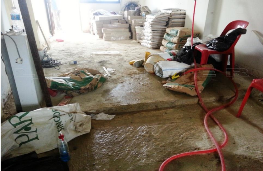
Before application, recessed at kitchen area
