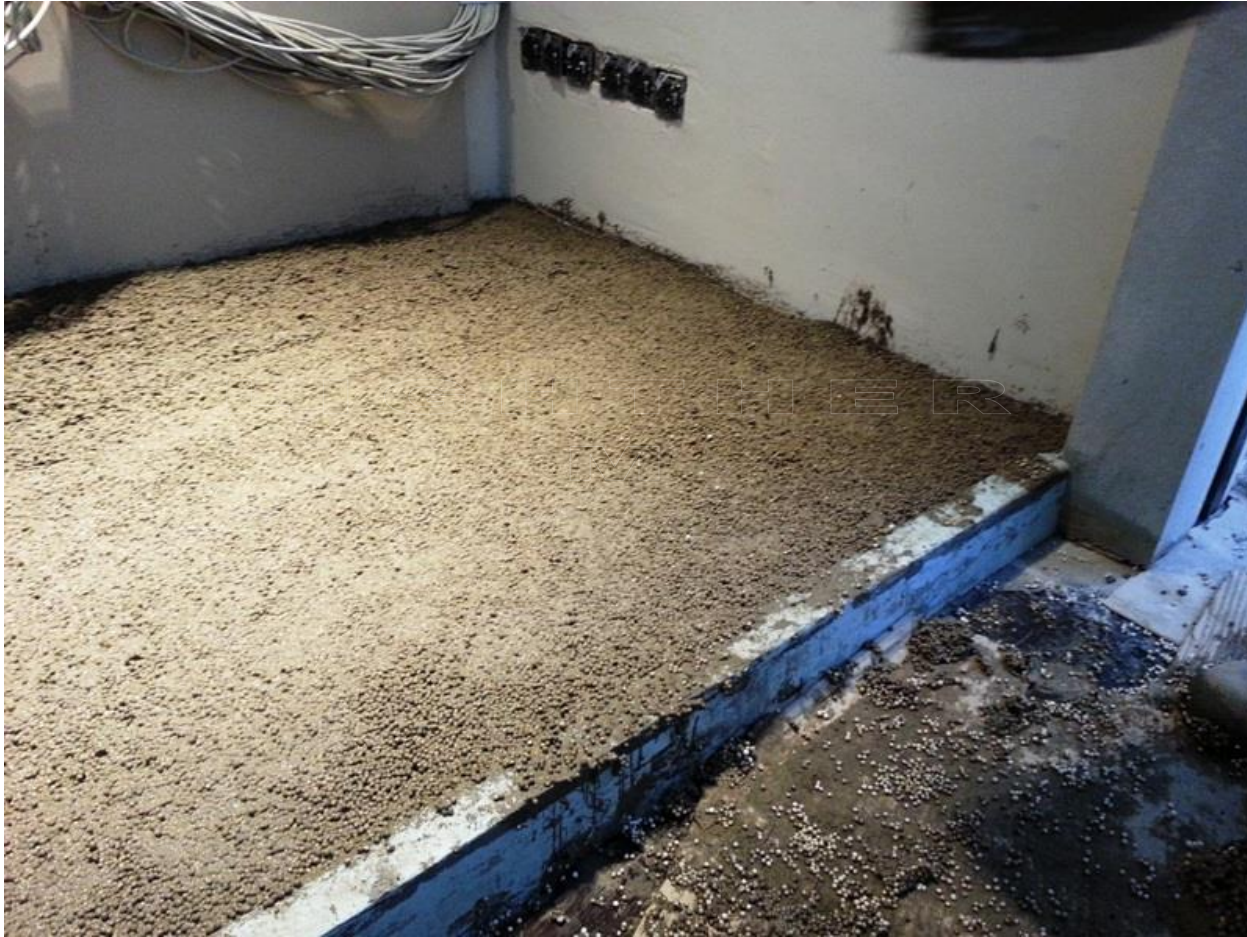
Insulation layer to prevent condensation -- Conservation Unit @ 136 & 138 Neil Road
