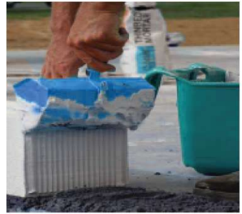
Figure 5D.3: Applying VODAPRUF ALC Block thin-bed mortar to vertical joint with notched trowel
