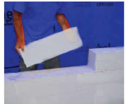
Figure 5D.8: Laying block by first setting backside down, then butting face of block is set into position
