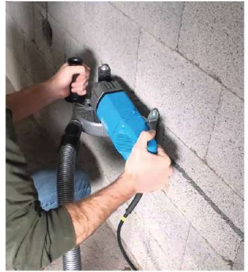
Figure 5D.13: Cutting chases into ALC wall
