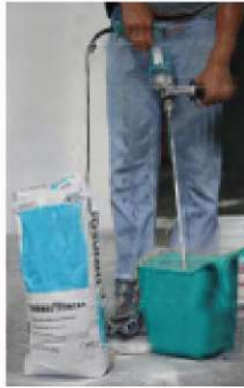
Figure 5D. 2: Mixing thin-bed mortar
