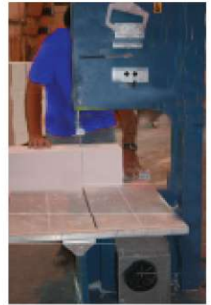
Figure 5D.5: Cutting ALC with band saw
