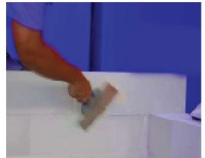
Figure 5D.9: Removing spilled mortar from joints
