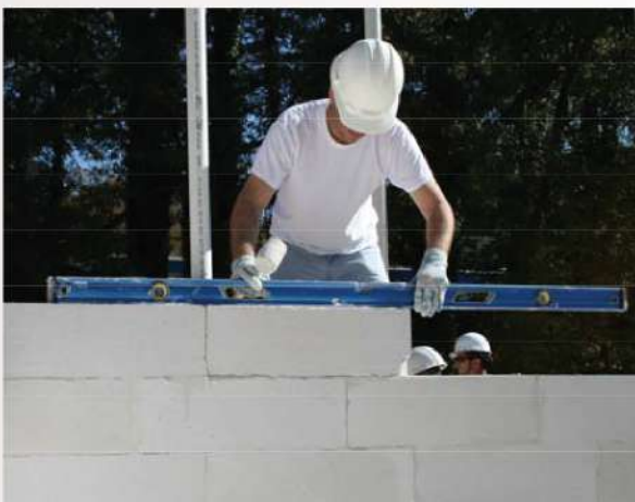
Figure 5D.10: Checking alignment and level of wall
