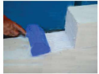
Figure 5D.7: Applying thin-bed mortar on horizontal joints
