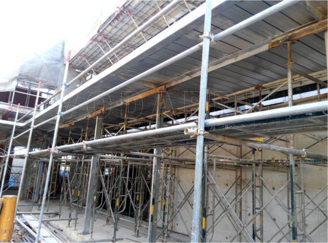
Bondeck ( Steel Decking)
