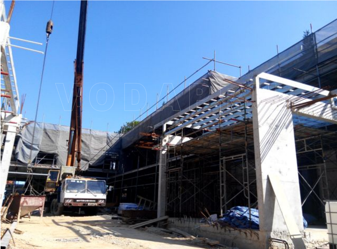
Lightherm being hoist up
