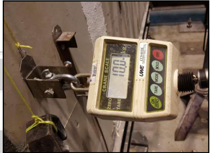
Figure 18 : Lightweight anchorage- pull-out test
