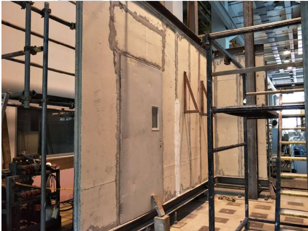
Figure 3: Test specimen mock-up
